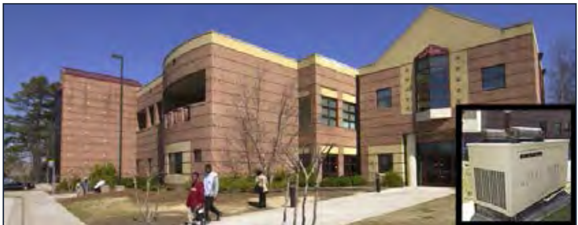
Establish at least one alternate storage facility where vaccine can be appropriately stored and monitored. This facility should have a back-up generator.
